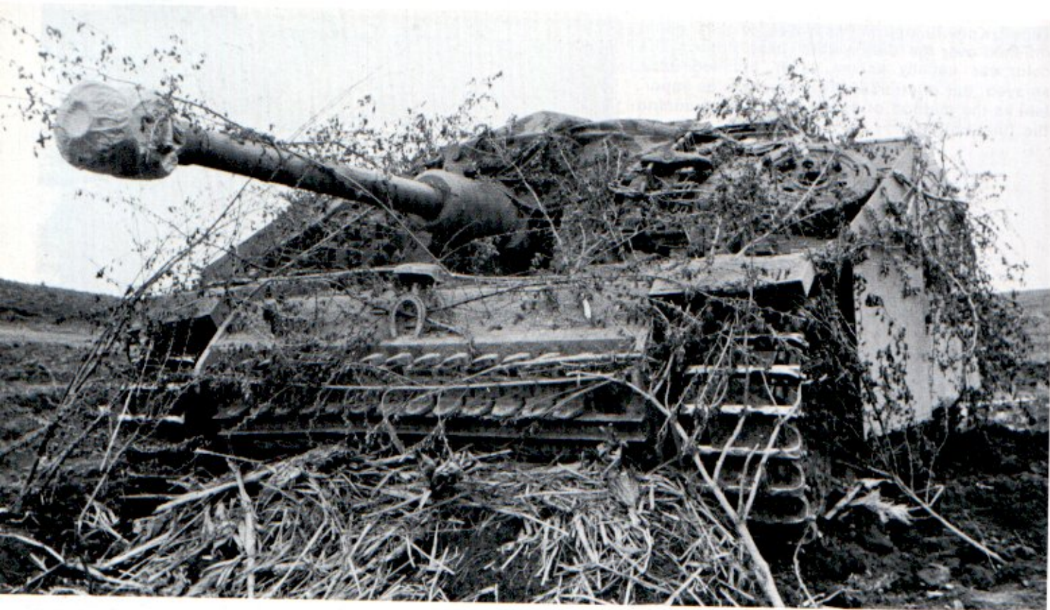
A StuG III ausf G in overall dark yellow, in Russia, 1943. There are no second colors applied, and the main camouflage is provided by the foliage piled around the vehicle. A camouflage tarpaulin is spread on the roof for more effective concealment.
