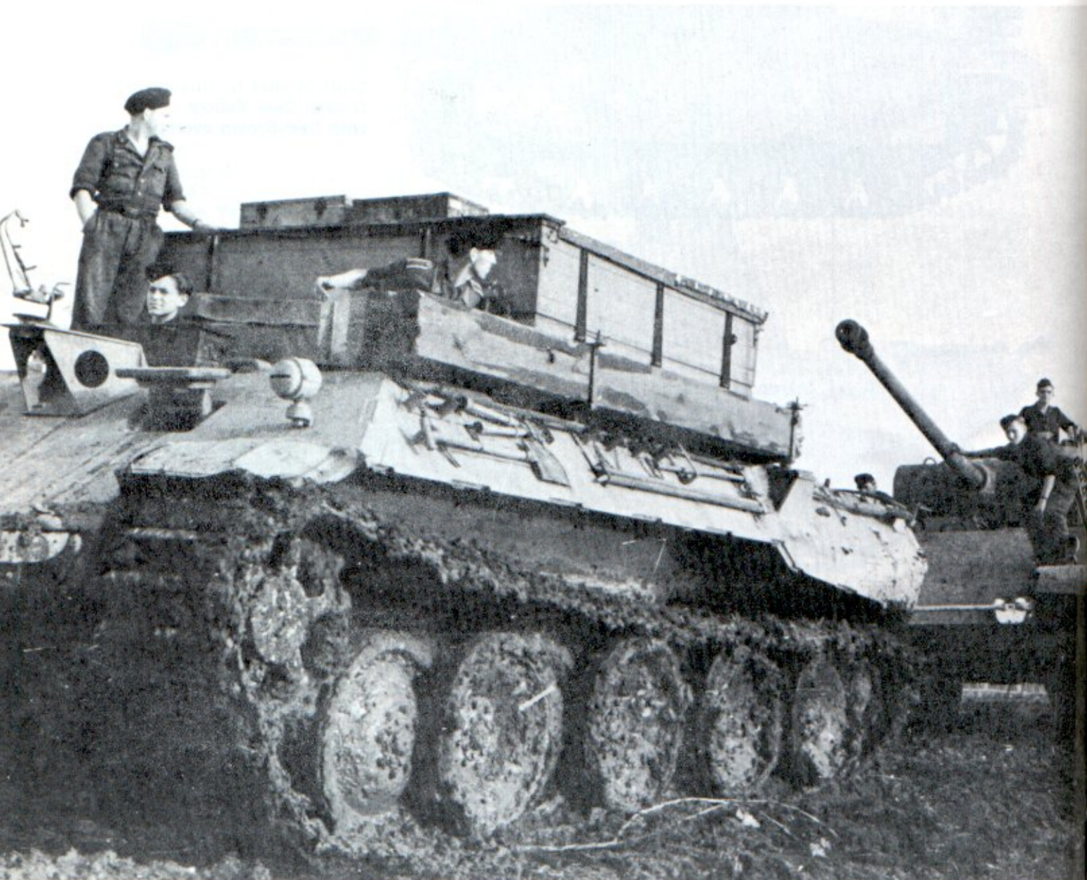
A Bergepanther recovery vehicle tows a disabled Panther ausf G. Both vehicles are dark yellow. Note the tow hook at the front of the Bergepanther - two vehicles are towing the Panther. An anti-aircraft MG mount has been attached to the base for the jib, on the glacis plate. [Bundesarchiv]
