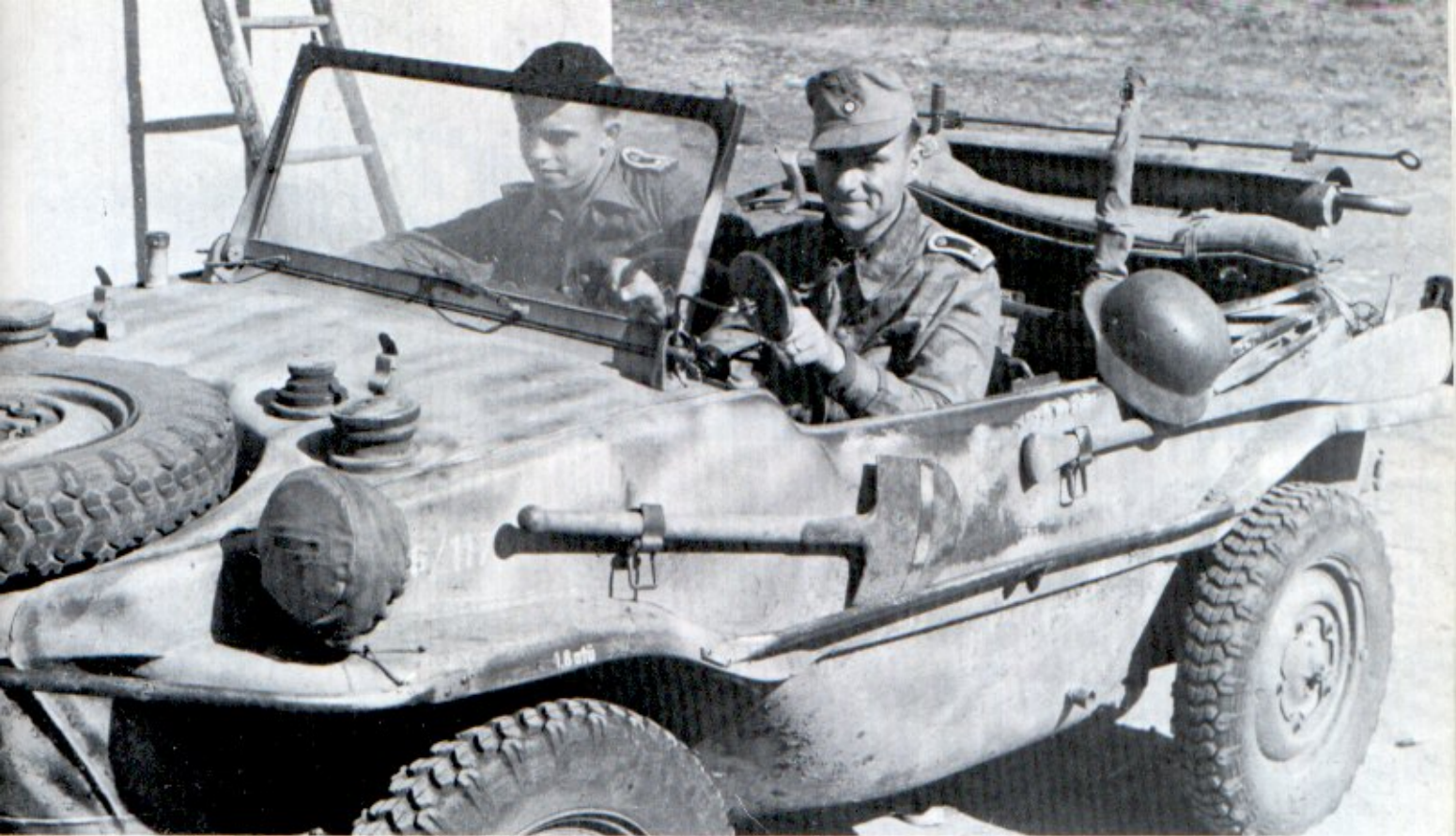
A Schwimmwagen in Russia, showing an extensive sprayed pattern of dark yellow over the dark gray. The yellow has been work away from the upper edges of the body. Paint was often rubbed off corners or protruding structures. [Bundesarchiv]
