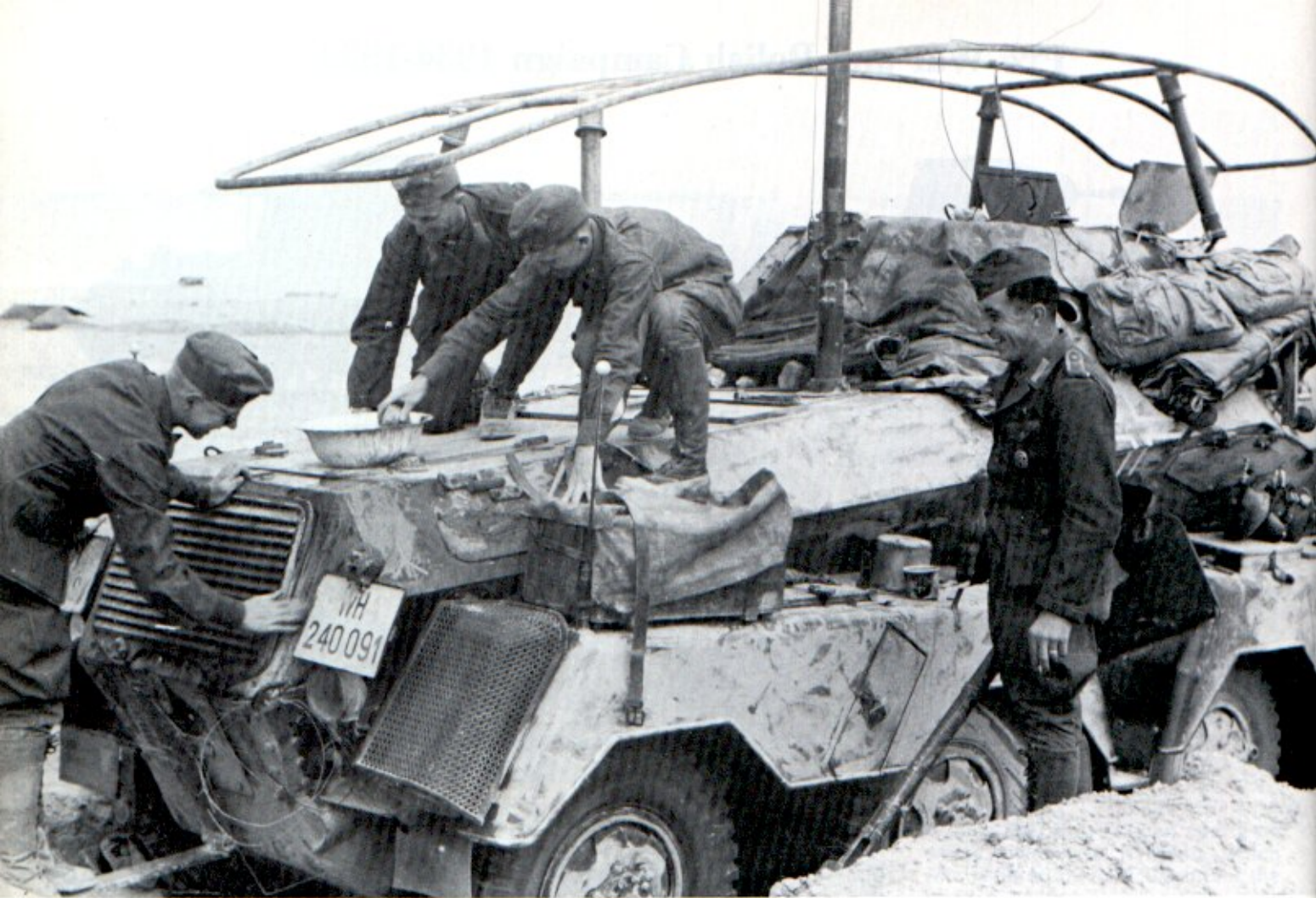
The crew of this SdKfz 263 armored car applies soupy mud to the rear deck and sides. When dry, the mud will match the rest of the vehicle, already covered with mud.
