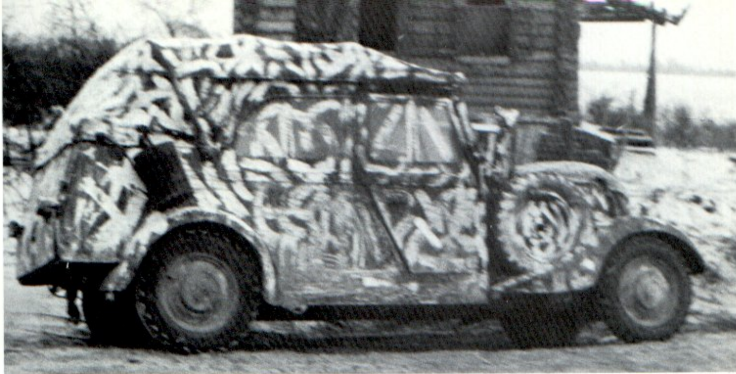
The supplies of white paint and even calcimine whitewash were often limited, and crews had to stretch the amount by painting only parts of the vehicles or by use of patterns of stripes or spots in white. [Bundesarchiv]
