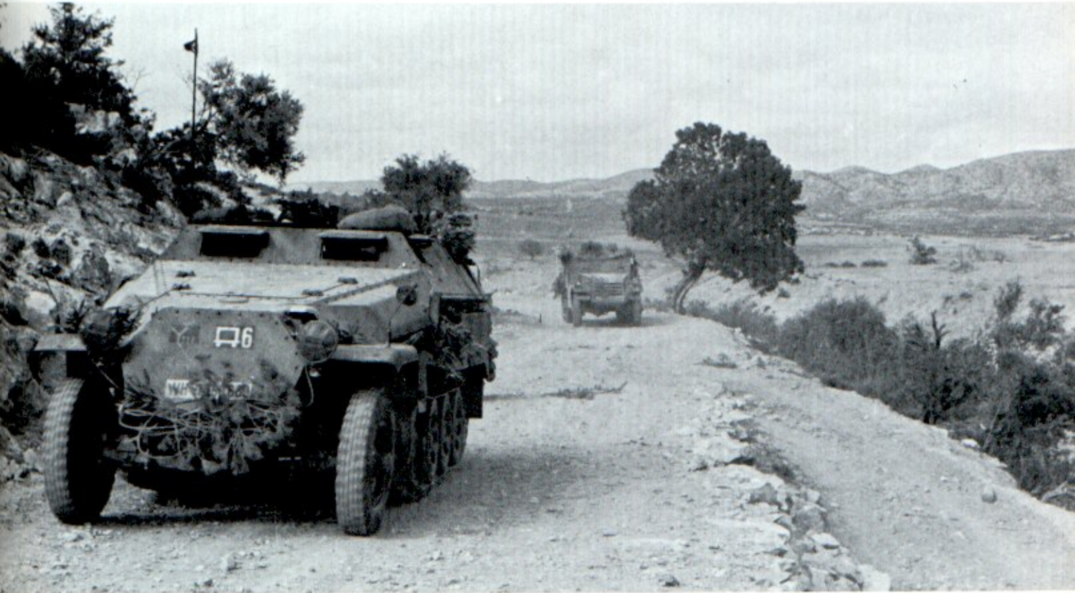
A SdKfz 251/1 ausf C [s.MG] leads a captured U.S. M3 halftrack down a road in Tunisia. The SdKfz 251 is from the 10th Panzer division, and has been repainted with an overspray of dark yellow covering the dark gray base. The insignia have been masked off, as was common early in the African campaign. [Bundesarchiv]
