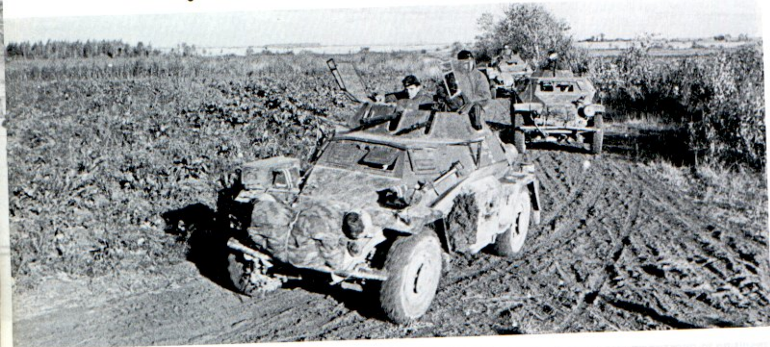
This early SdKfz 222 armored car, followed by an SdKfz 223 and an SdKfz 221, in Russia during mid-1941 show the effects of heavy mud on vehicles. Thick wet brown mud is still clumped on parts of the vehicles. Dried mud is much lighter, and covers virtually all of the vehicles' lower hulls and chassis parts. [Bundesarchiv]
