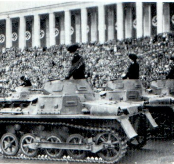
PzKpfw I ausf A's at a Nazi rally in 1934, showing the use of the Reichswehr colors in 3-color sprayed "cloud effect" schemes. The lead tank has a pennant.
